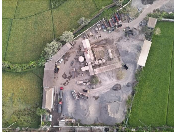
Figure 1. Existing Work Area
